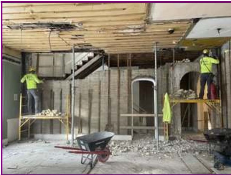
Workers remove bricks, one at a time, from the monastery.
