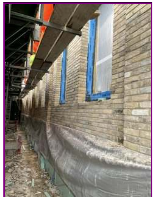
North wall of the new parish center.
